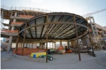
The ballpark's Vertical Circulation building, still under construction.
