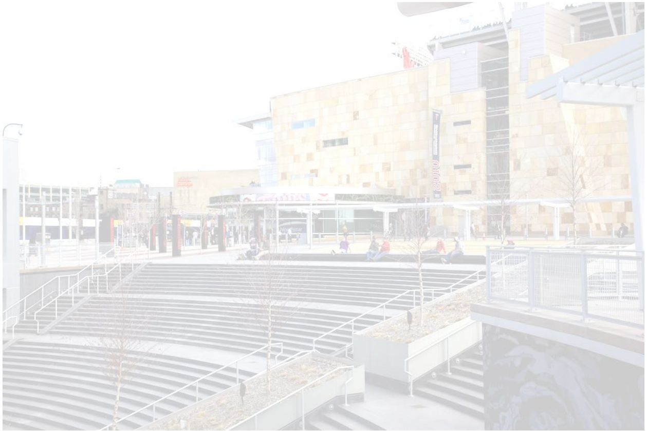
MINNESOTA BALLPARK AUTHORITY Hennepin County, Minnesota
